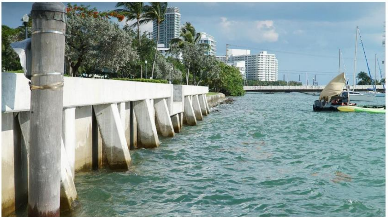
Figure 16: Seawall in Miami beach (USA)
