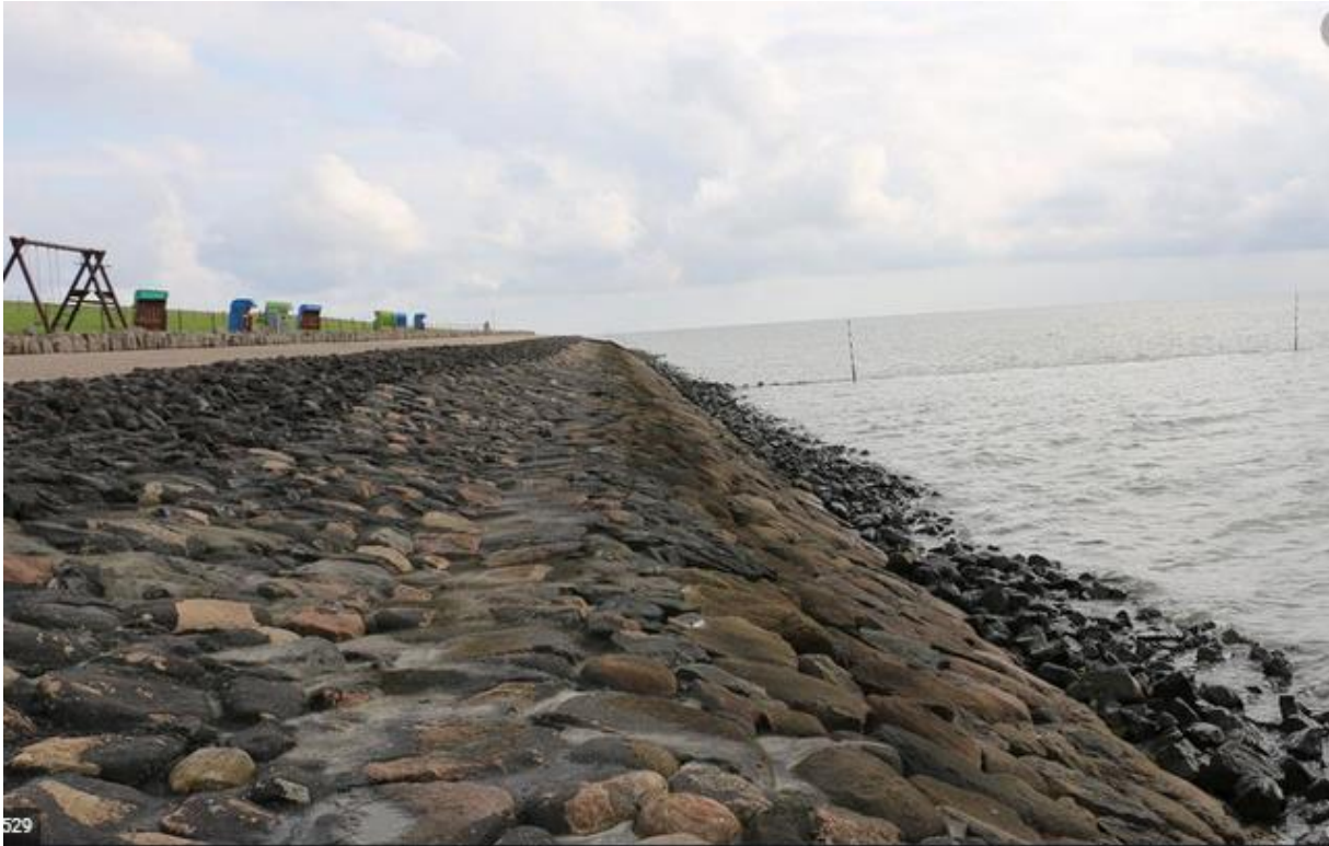
Figure 17: Example of a dyke in German island of Pellworm
