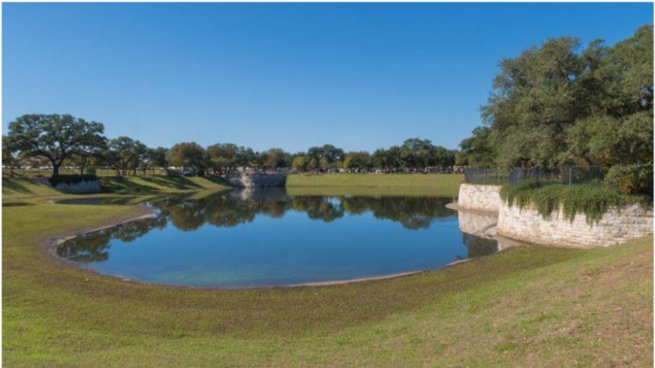
Figure 33: Example of retention and filtration pond near Berlin
