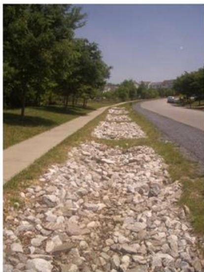
Figure 28: Example of system to collect runoffs from impervious surfaces such as roofs, walkways and parking lots and infiltrate it into the ground in urban areas (infiltration trenches and rain garden) ( Technical Training Manual on Urban Circular Water Management for Municipalities – Association for Rainwater Harvesting and Water Utilisation – INTERREG project – 2019 )
