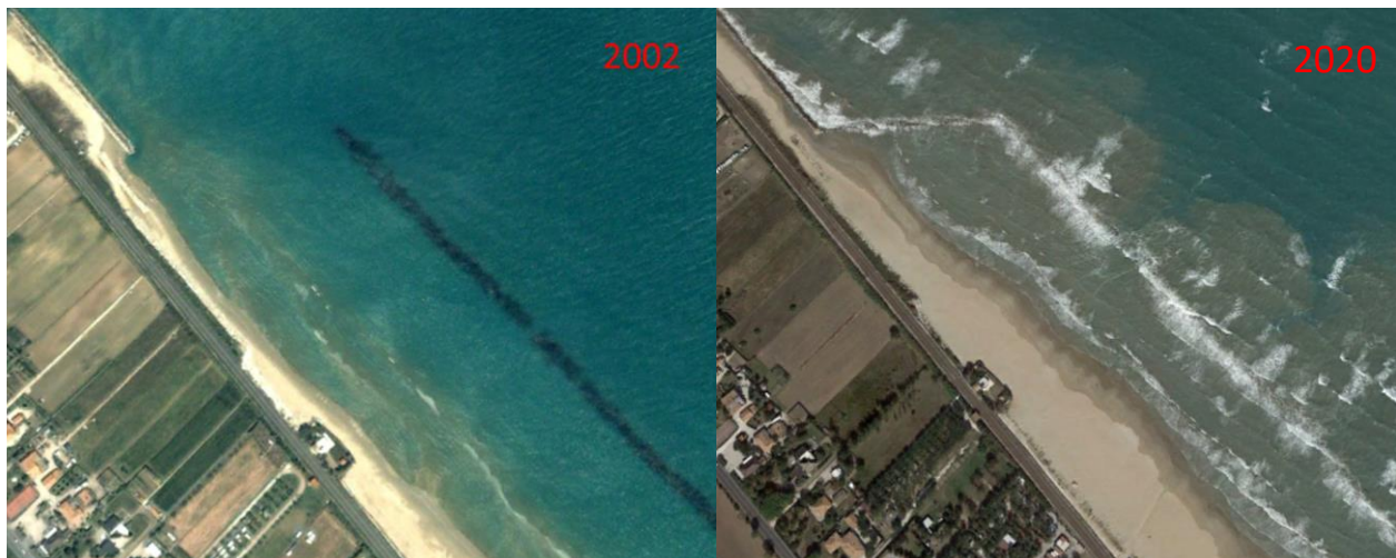
Figure 14: Artificial reef offshore breakwater at Fano in 2002 and in 2020
