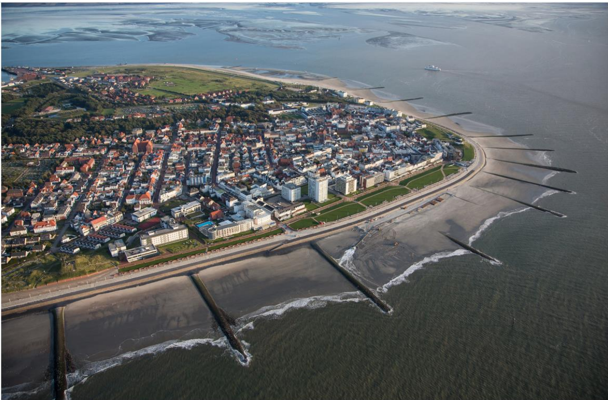
Figure 15: Rock groynes in Netherlands
