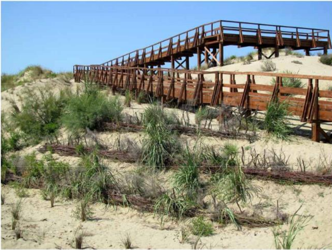
Figure 18: San Rossore dune with wooden pedestrian walkway and revegetation with pioneer plants (Boccalaro, 2008)
