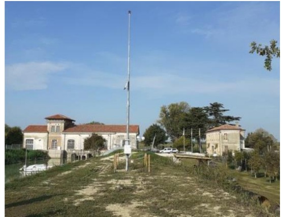
Figure 2.3-23 View of the new station towards the West (drainage plant and guardian house).
