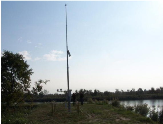
Figure 2.3-22 View of the new station towards the East (Desse River can be seen)
