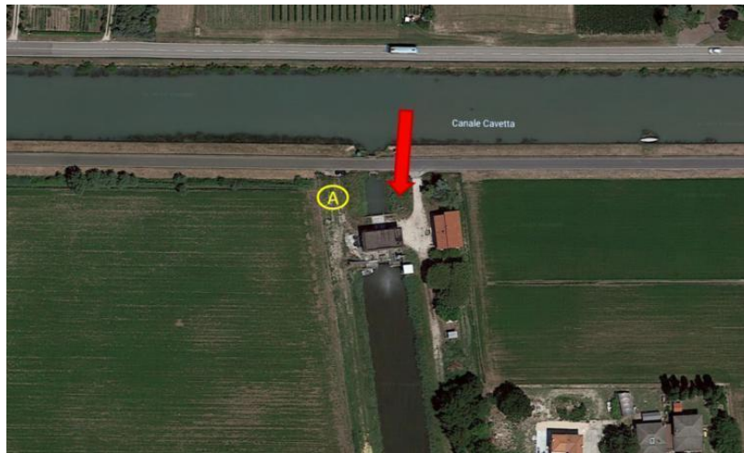
Figure 2.3-11 Aerial photo of the dewatering plant; The red arrow identifies the site of the historic station, the yellow circle identifies the site of the new station.
