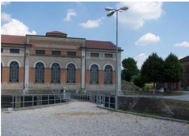
Figure 2.3-3 The dewatering plant and the historic station on the right
