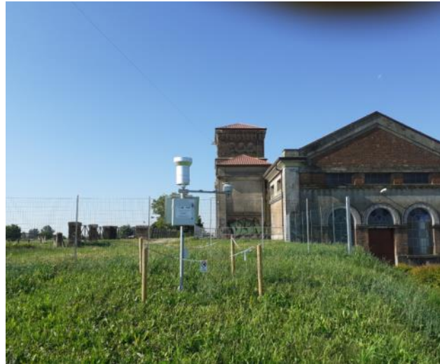
Figure 2.3-6 Station view from the North
