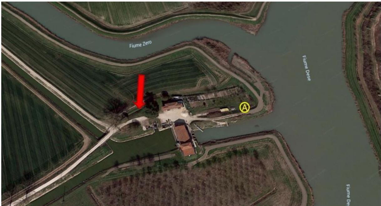
Figure 2.3-19 Aerial photo of the drainage plant located near the confluence of the Zero and Dese Rivers; the red arrow identifies the site of the historic station, the yellow circle identifies the site of the new station.
