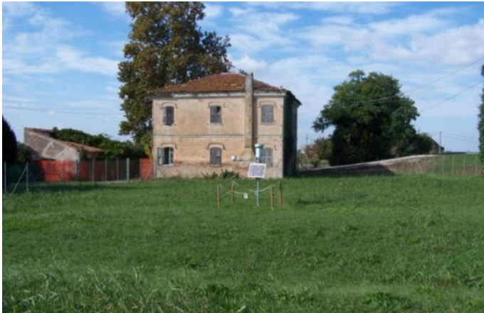
Figure 2.3-30 View of the new station from the South-East
