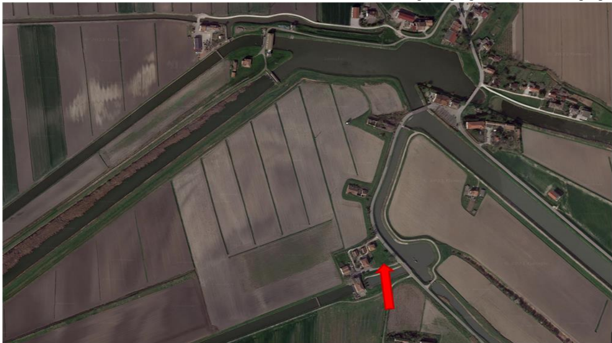
Figure 2.3-29 Aerial photo of the dewatering plant. The red arrow identifies the site of the historic station which is exactly the same as the new installation. Towards the North there is a second drainage plant named Santa Giustina.
