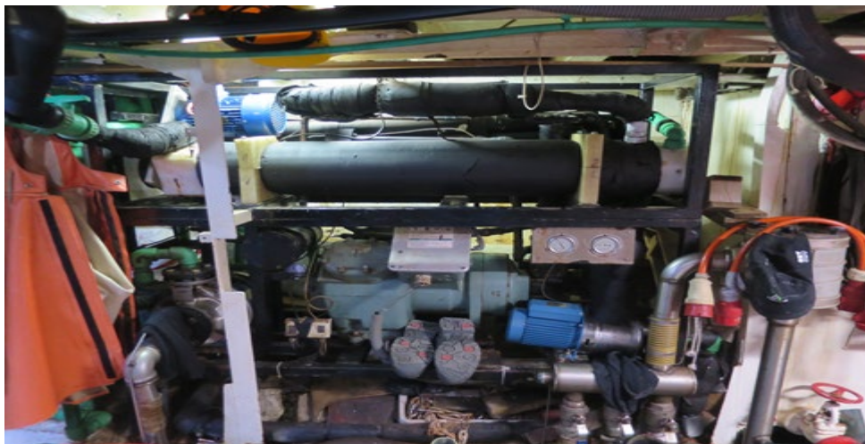
Figure 20. Plant for the production of a mixture of cold sea water and ice on board B (source: WWF
