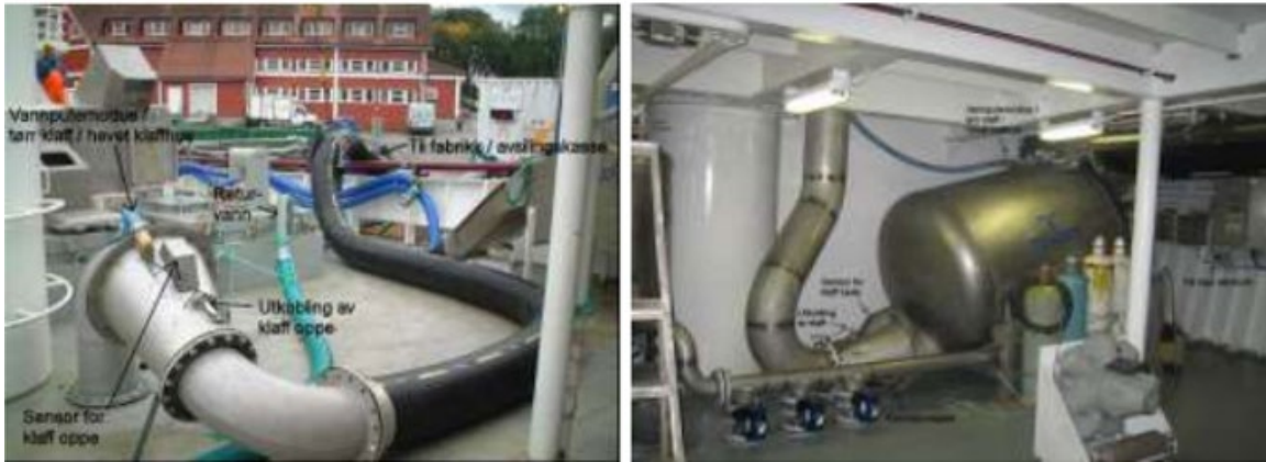
Figure 24. The space needed for high-dimensional pumps tanks and pipes (Source: Aursand G et al., 2011-SINTEF-Norway)
