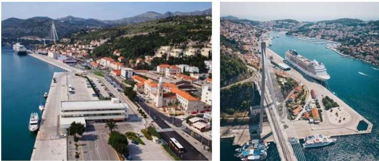
Figure 1: Port of the city of Dubrovnik existing situation
