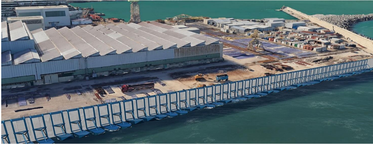
Figure 26 - Birds'eye view from the sea of the power plant
