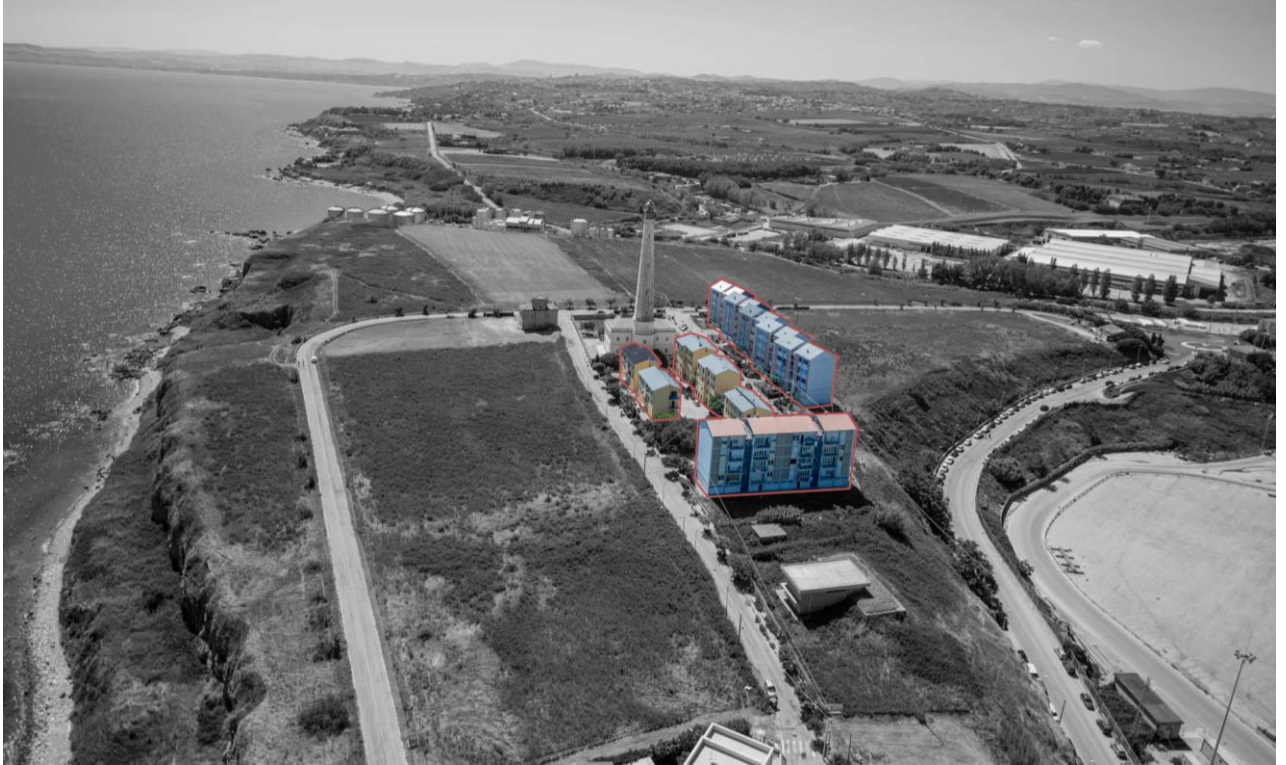
Figure 8 - Buildings for heat pumps installation (about 10.000 m 3 ). Image source: ASPO Ortona and Vasto website.
