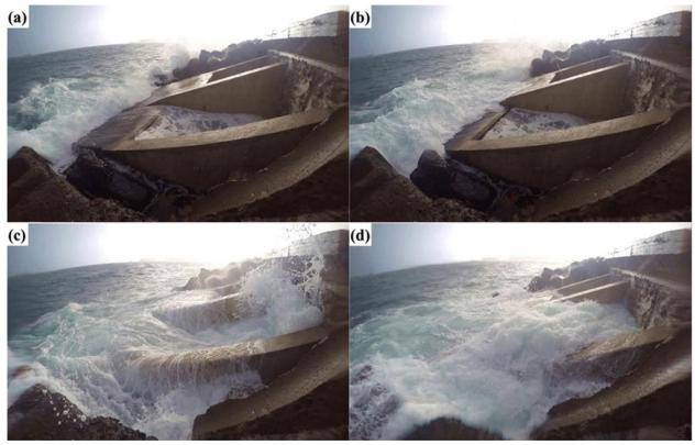
Figure 53 - OBREC device in operation.
