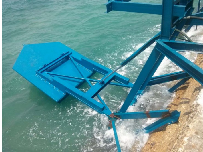
Figure 40 - Installation of EWP converters at Jaffa port [20]
