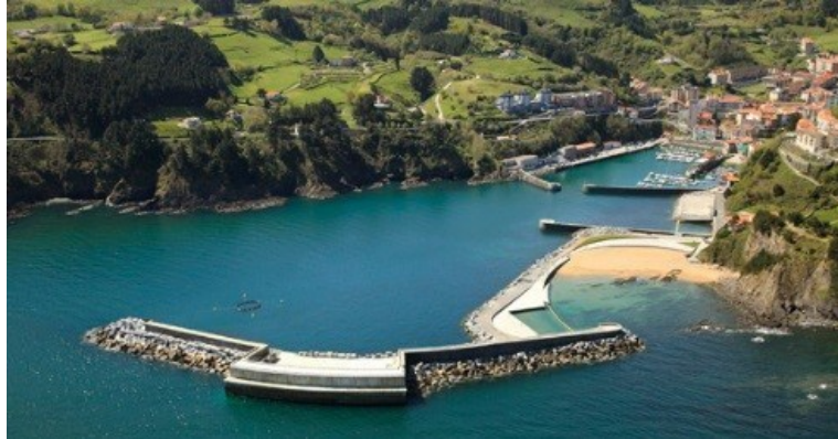
Figure 39 - Breakwater with installed wave energy converter in Mutriku [19]
