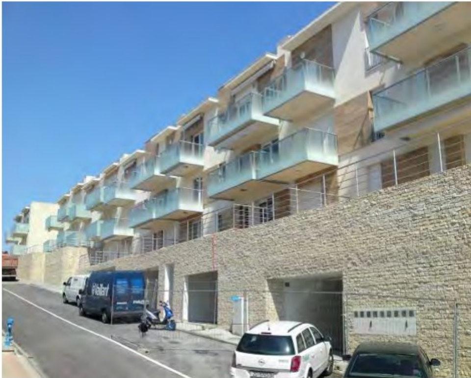
Figure 46 - The apartment building, Pazdigradska ulica, Split
