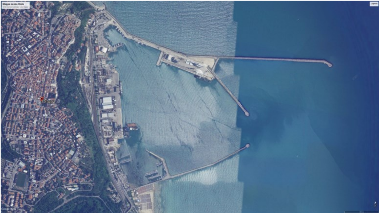
Figure 105 - Port of Ortona: current state
