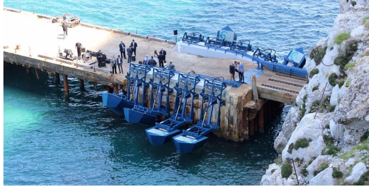
Figure 31 - Wave clapper installed on an existing structure (Gibraltar – EWP)
