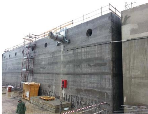
Figure 3 - Work in progress
