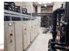
Knežev dvor, new facilities
