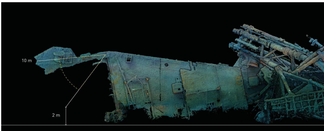
Figure 2: part of the Paguro wreck that was fallen apart during the 2021 winter period.
