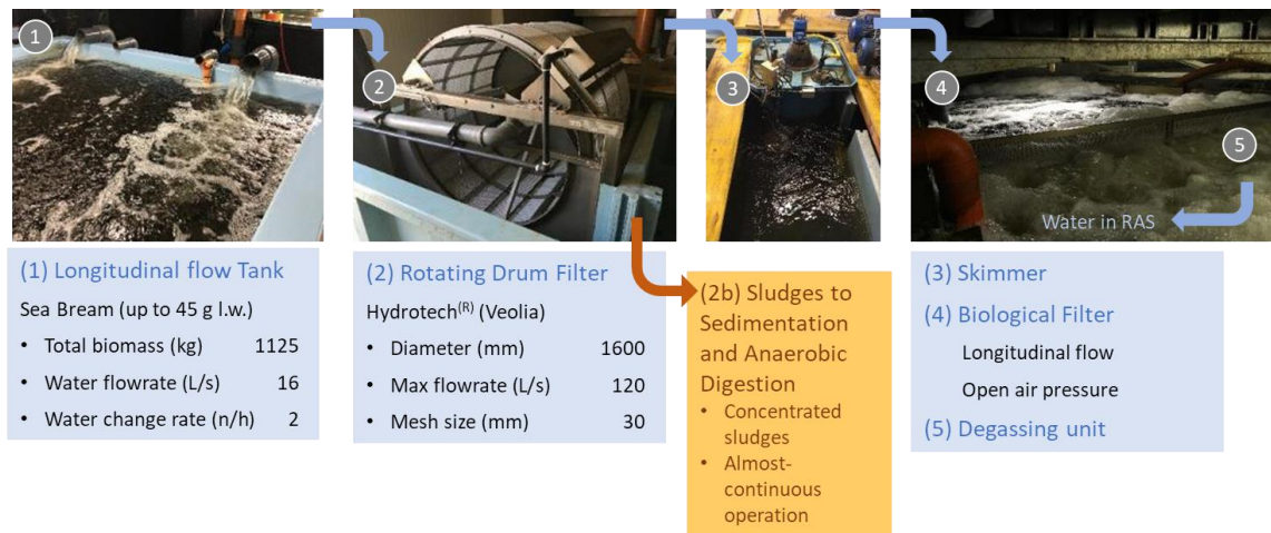
Figure 3. Layout of the recirculating aquaculture system (RAS) installed in PP9 fish farm.
