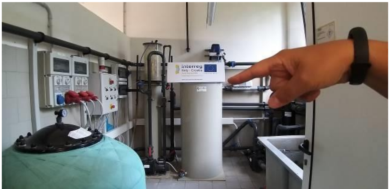
The white cylinder in the foreground is the biological filter, on its back a protein skimmer (or foam fractionator) to remove organic compounds from water of the RAS system.
