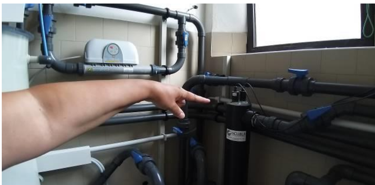
UV sterilizer lamp apparatus connected to the RAS system.
