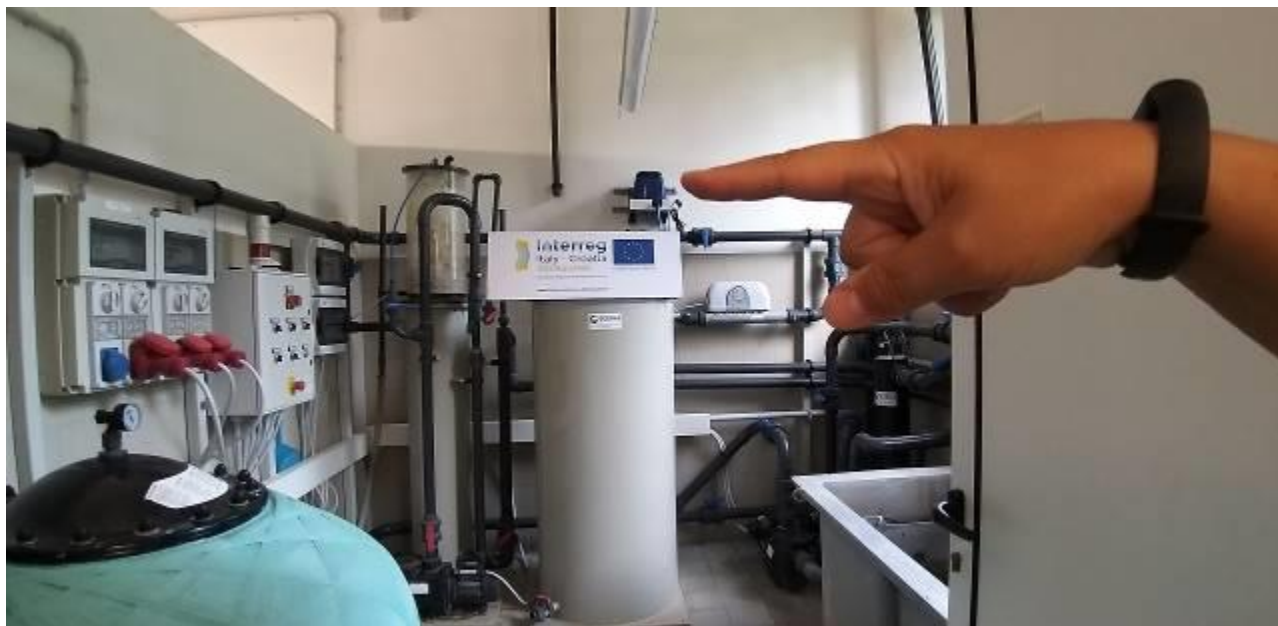
Ozonator for disinfection of waste water to be discharged from the RAS system.
