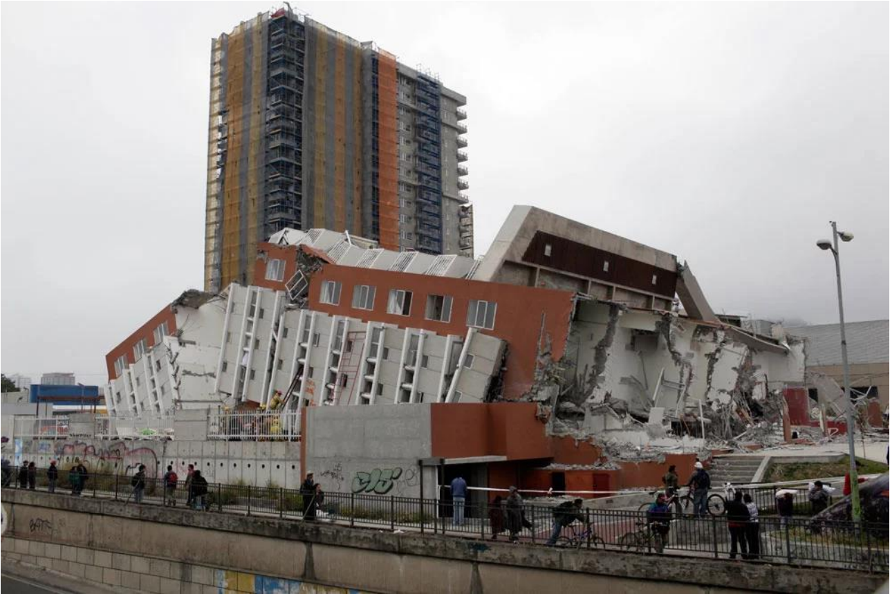
(Twenty five survivors have been rescued from this collapsed apartment building in Concepcion, Chile. Nine bodies were recovered. Natacha Pisarenko/AP Photo)
