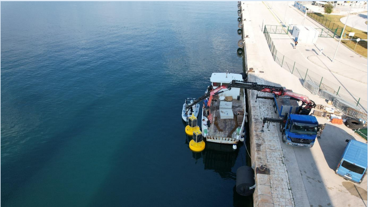
Figure 3. The process of placing and securing the buoy for transport to the anchoring location (photo made by air drone)
