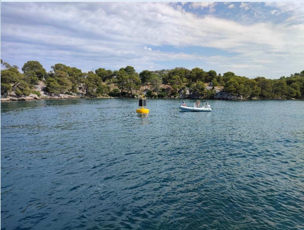
Figure 12. Installed second buoy on the other side of the entrance in a channel of st. Ante
