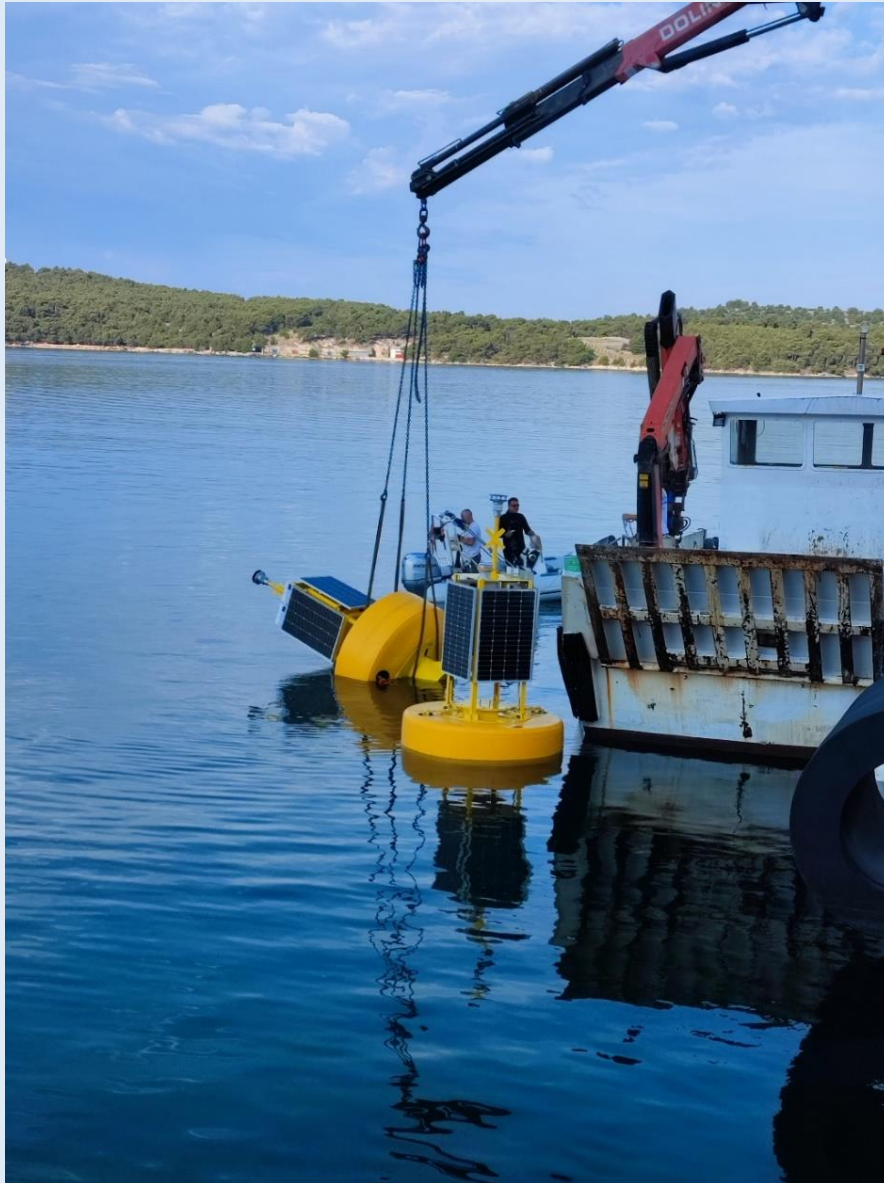
Figure 2. The process of placing and securing the buoy for transport to the anchoring location
