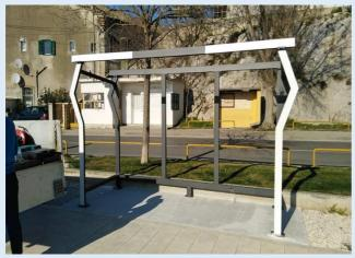
Small infrastructural works included the preparations of the concrete foundations and were finished in December 2020. Construction, placement and installation of the waiting stations started immediately after that.
