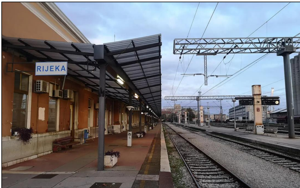
Figure 17. Rijeka Railway station
