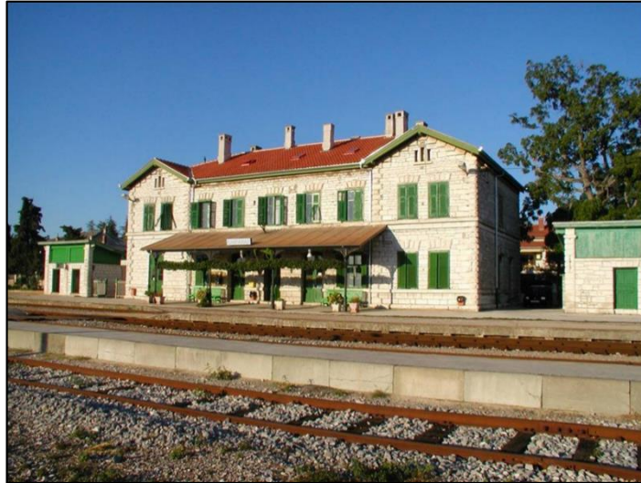
Picture 8. Interchange node in Kanfanar (bike/train connection from hinterland to coast)
