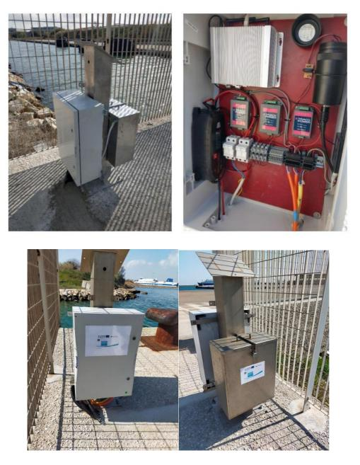
The probes and the power supply and data collection system are connected by 3 multi-conductor cables reinforced in kevlar, inserted in underground corrugations
