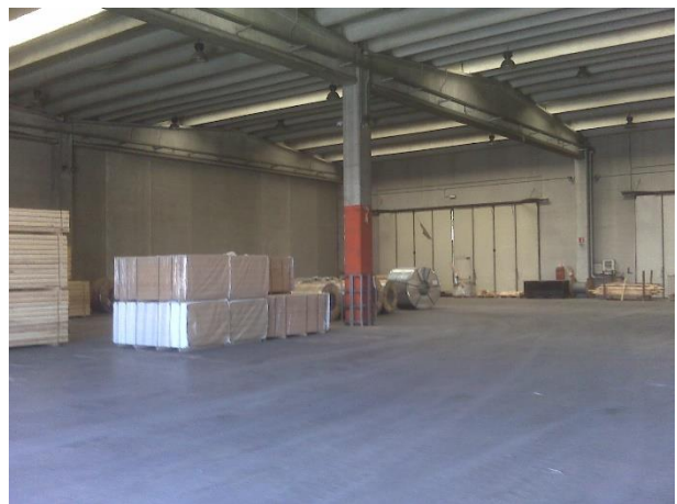
05 Port Warehouses Interiors
