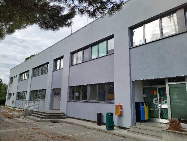
06 Service Building exteriors
