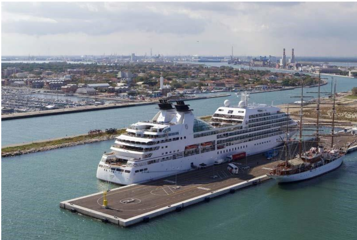
Figure 3: Site of the future cold ironing facility
