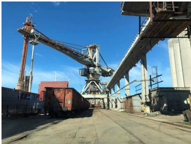
Figure 17: Metal crane near Silos
