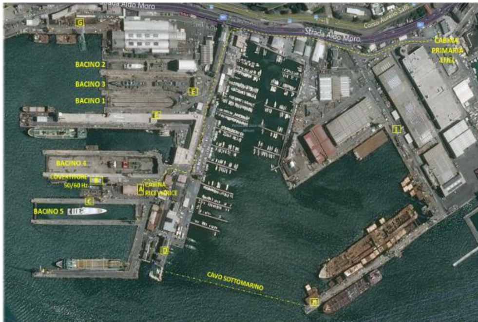
Figure 6 - Bacini di Carenaggio in the port of Genoa (Source: Port System Authority of the Western Ligurian Sea)
