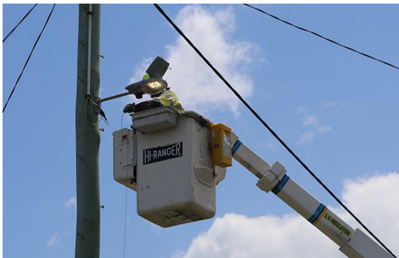
Figure 13 - Lighting system upgrade operations in the Port Macquarie - Hastings
