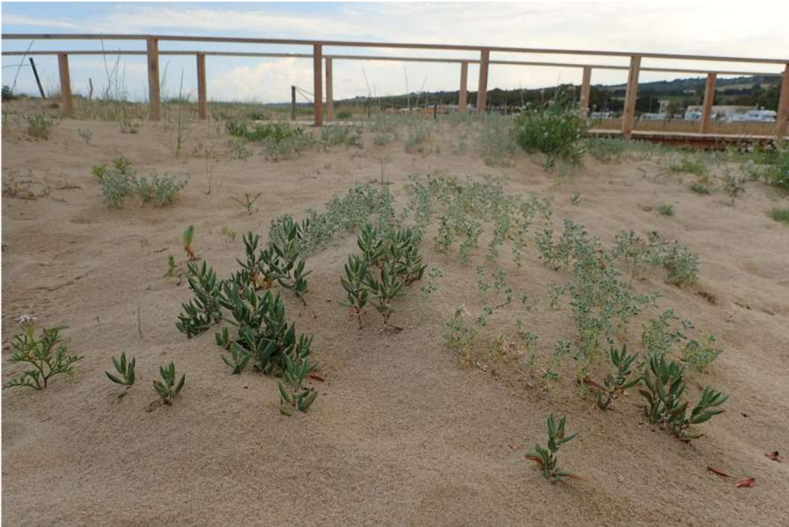
Fig. P2. 12. wooden broad-walk installed on central Adriatic coast for protecting sand dunes from trampling and for aiding nature to re-establish the natural dune coastal zonation.
