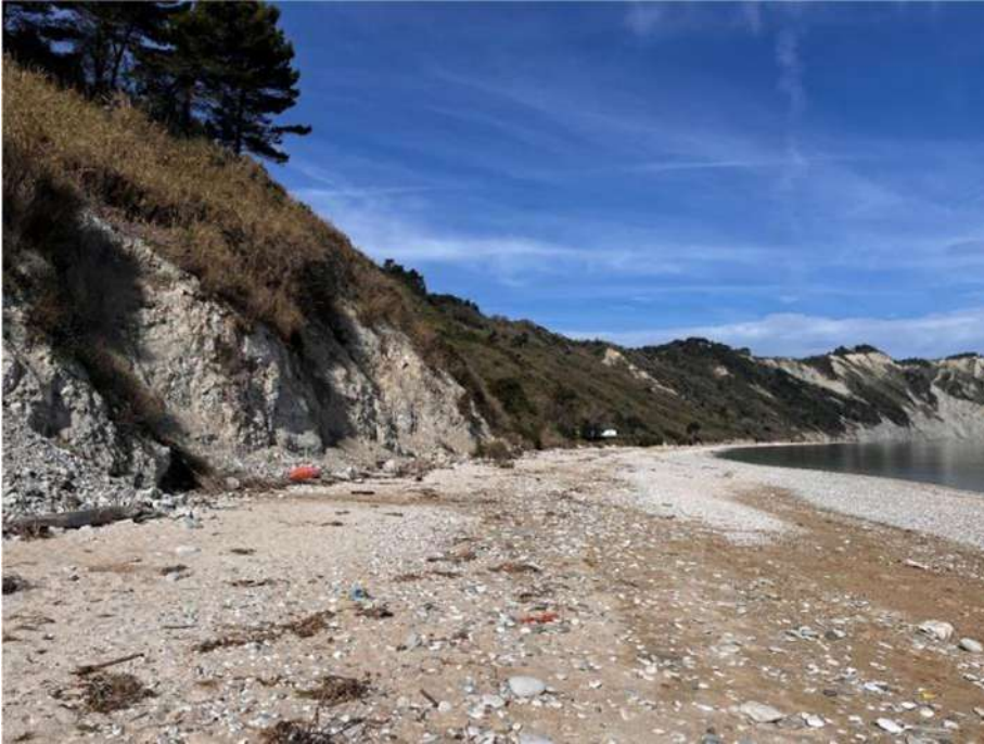
Figure 71. Transept 15_he_404 - Landslides and landslides of the upstream slope
