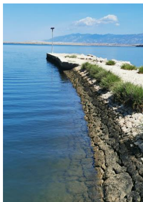
Figure 18. Inner side of the channel
