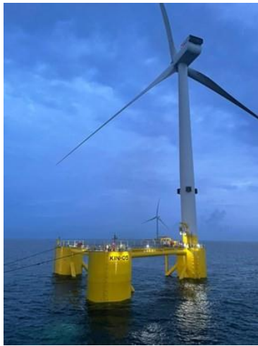
Figure 7 A floating offshore wind farm, Scotland, 2021
