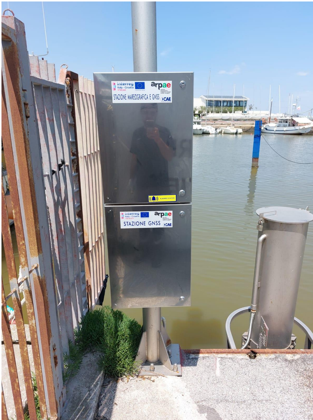
Figure 11. Picture of the tide gauge installed in Cervia (RA) with the logo
