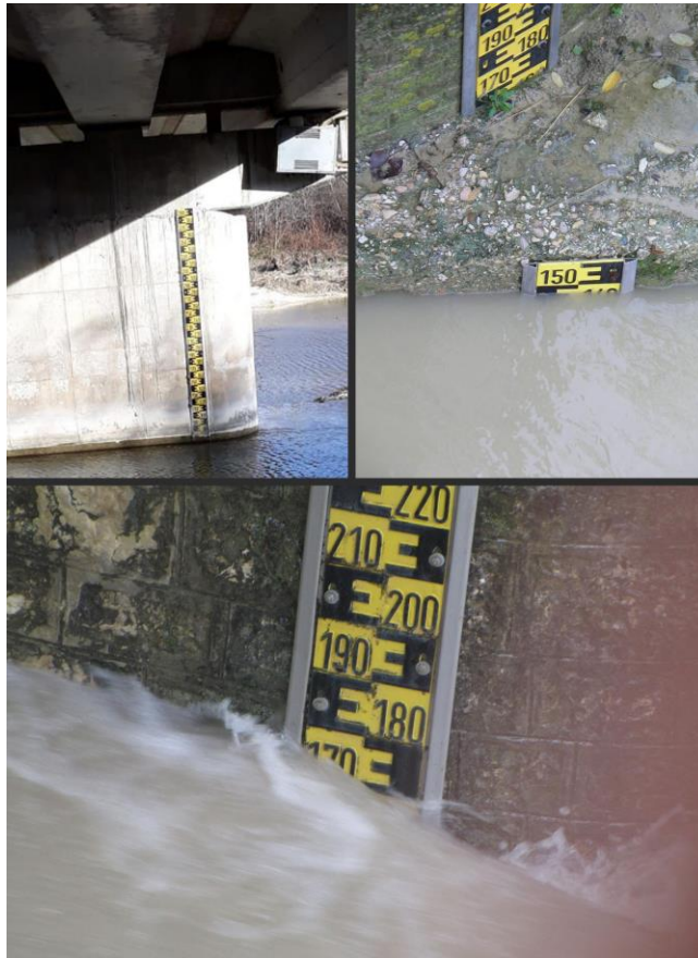
Figure 3: Example of hydrometric rod installed by the Civil Protection in each river
