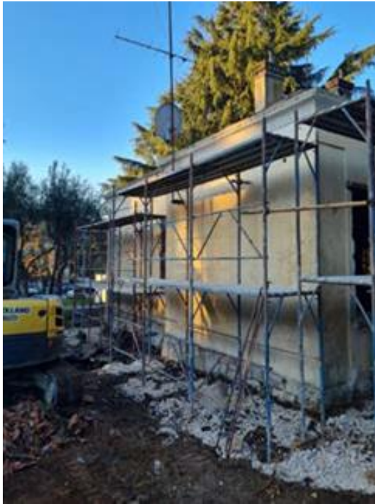
Works in progress
