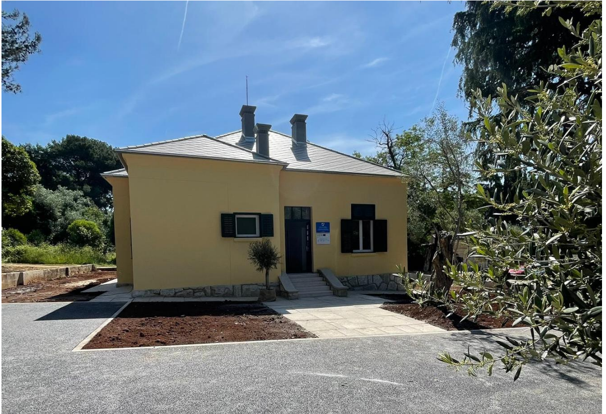
The Centre renovated
