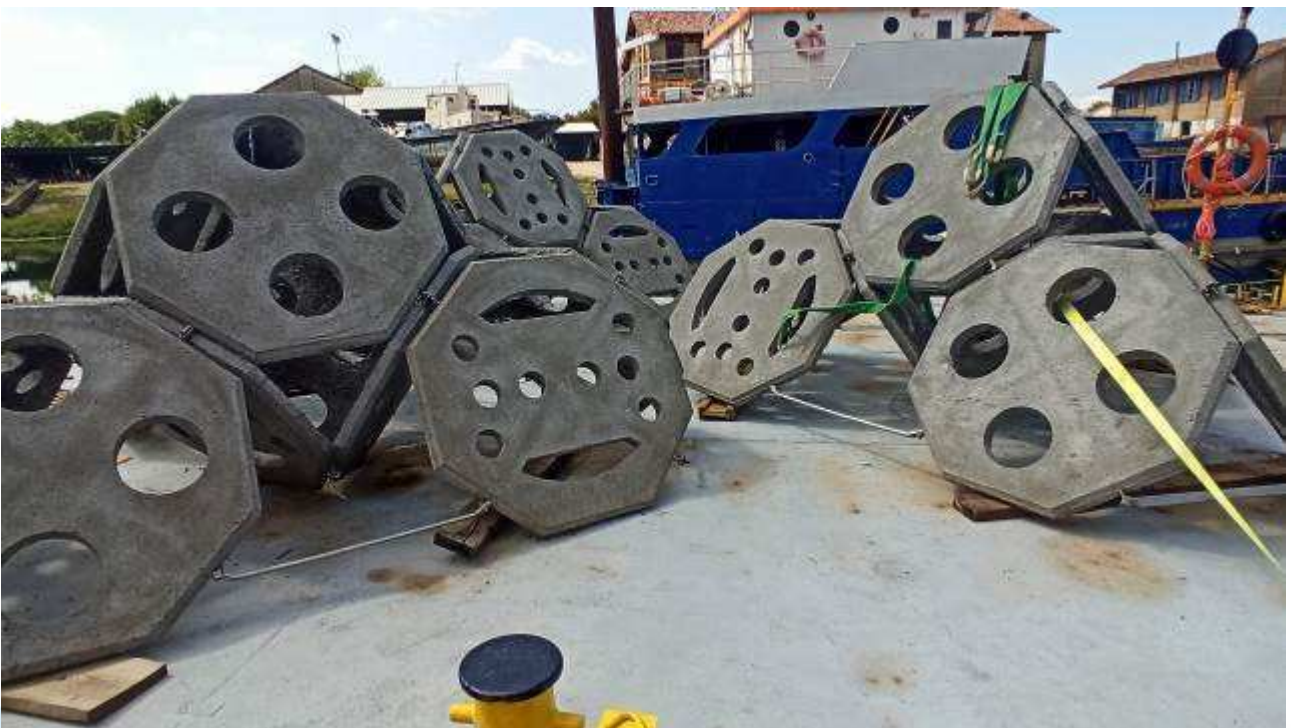
Photo 4: assembly of pyramid modules
