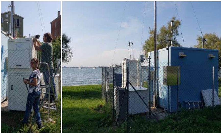
Figure 7.2. Details of the outdoor cabinet used for high-temporal resolution measurements.
