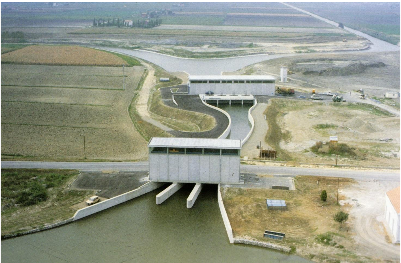
Drainage plant Nuovo Marozzo (1986)
