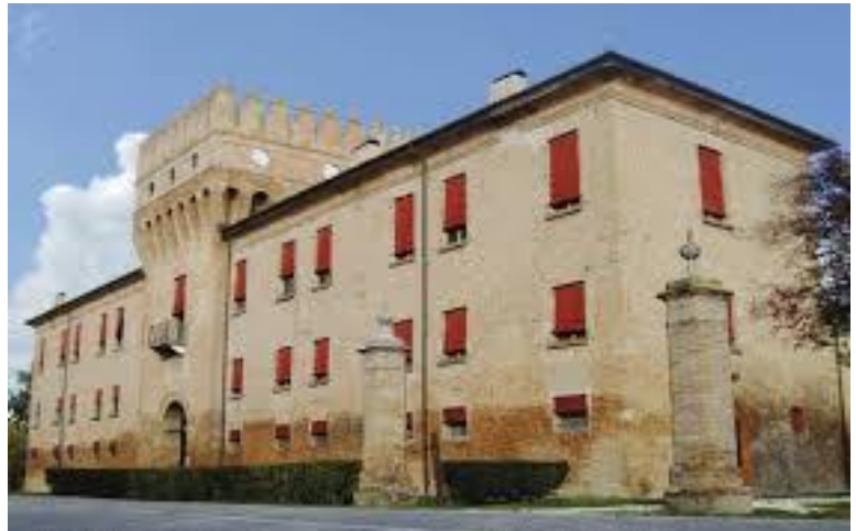
Main facade with tower
