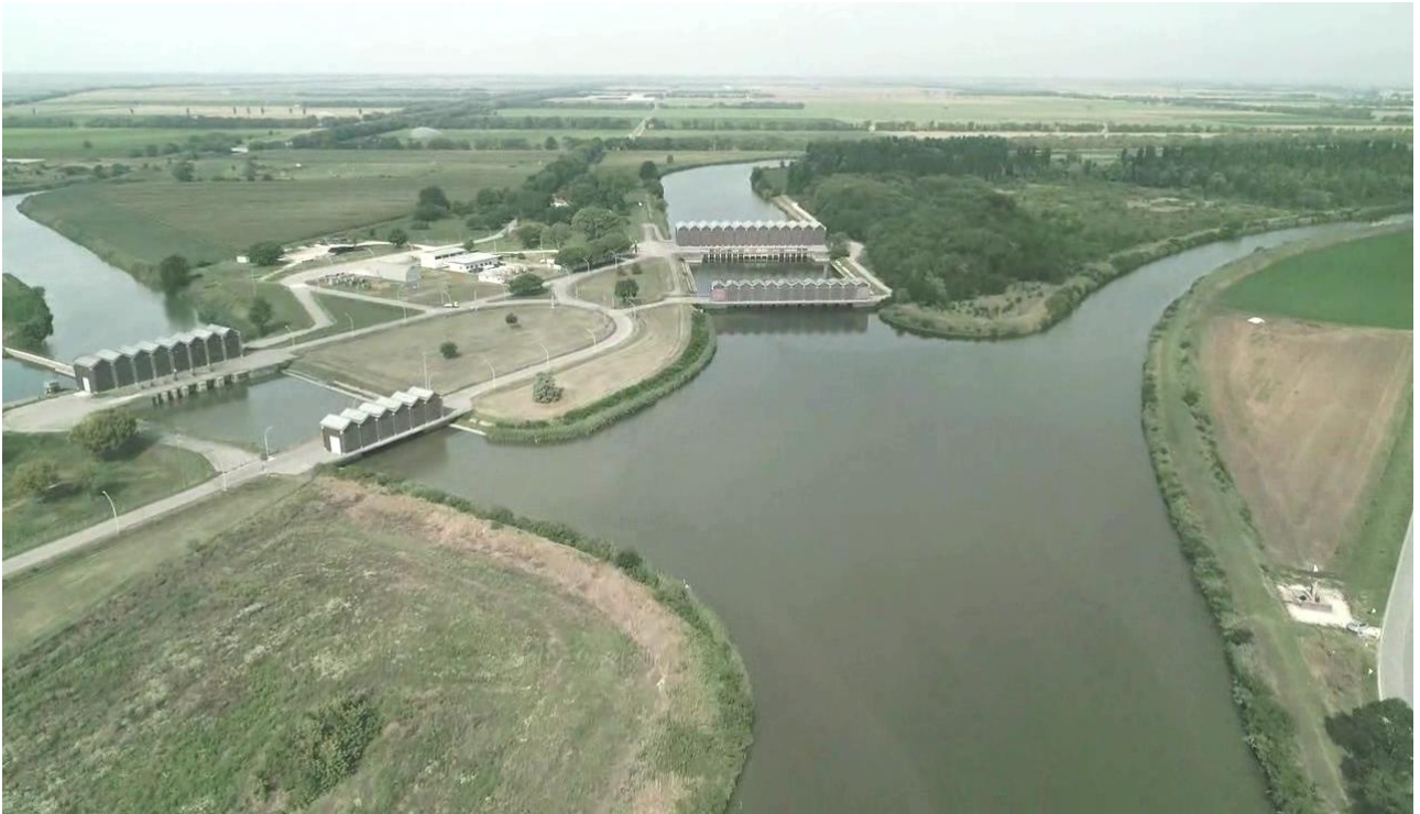
Drainage plant Lepri Acque Alte (is the largest hydro-drilling in Europe)
