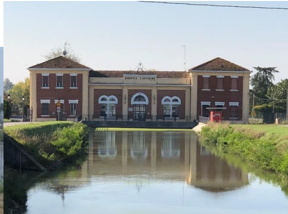
Drainage plant S. Antonino (1925), Ferrara
