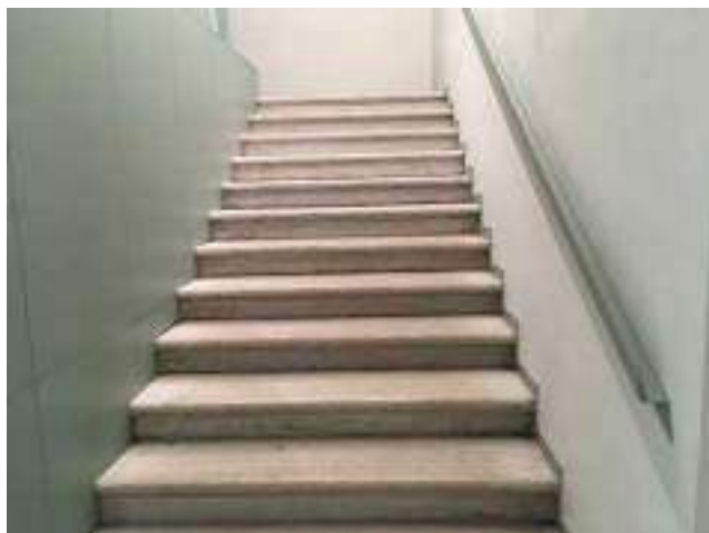
Fig.18 Connecting stairway between floors.
