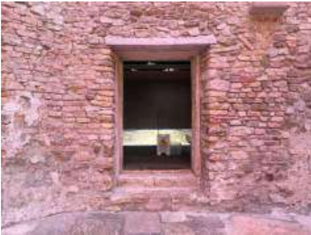
Fig.6 Internal view of the entrance from the Südhalle.
