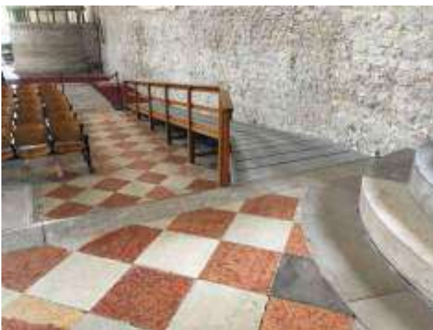
Fig.22 Wooden ramp with a railing at a height of 70 cm.
