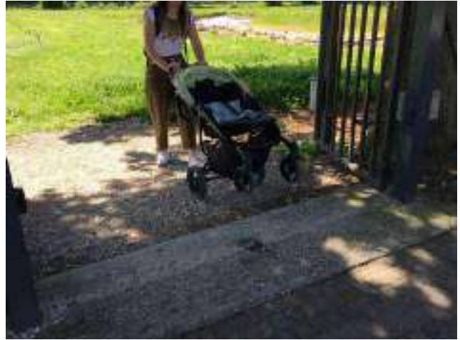
Fig.7 Necessity to lift up the pushchairs or prams to go beyond the obstacle.
