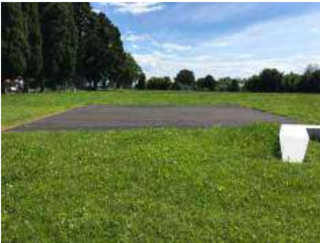
Fig.10 Platform in recycled material.
