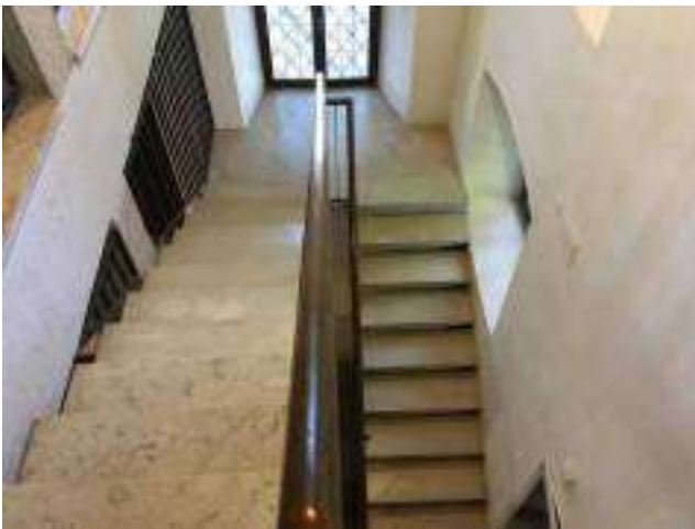
Fig.18 Linking stairs between the ground floor and the first floor.
