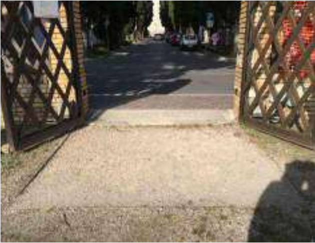
Fig.4 Internal view from the main gate.
