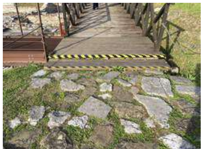
Fig.7 Final tract of the wooden walkway with security signage.
