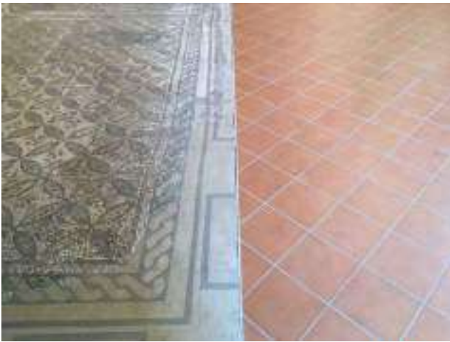
Fig.12 Paving in earthenware tiles with mosaics.
