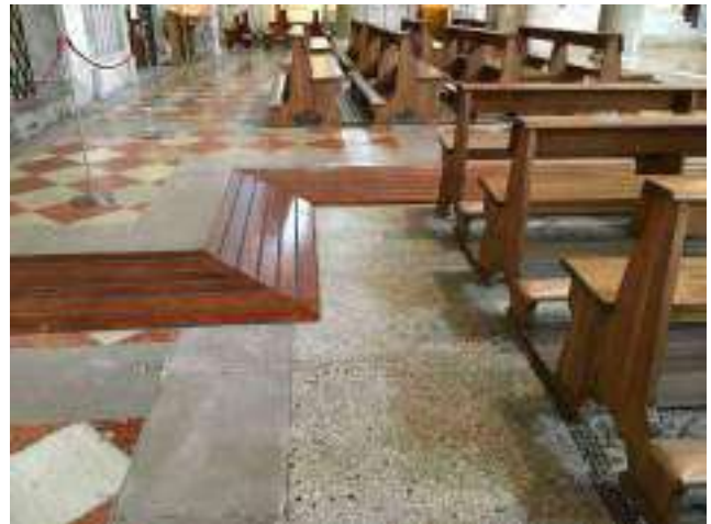
Fig. 17 Connecting wooden slopes.
