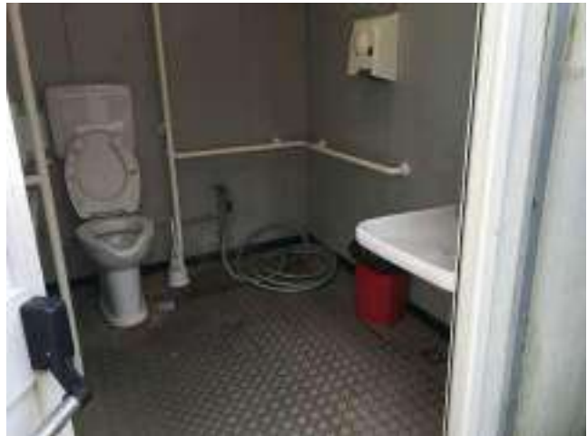
Fig.33 Toilet for the disabled
