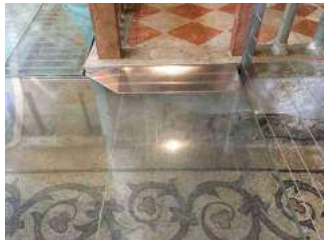
Fig.11 Metal ramp connecting the levels.
