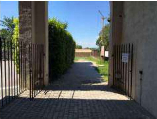
Fig.4 External view of the Southern entrance.
