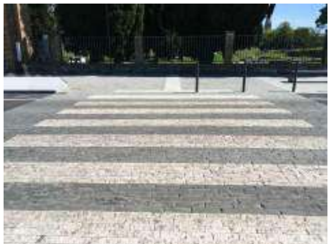
Fig.5 Pedestrian crossing with a tactilo-plantar loges.
