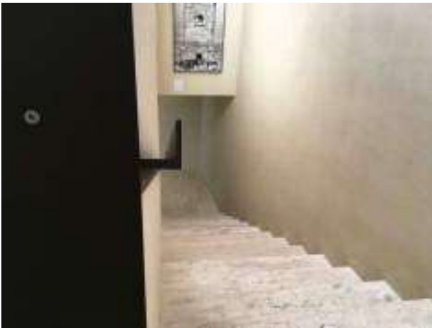
Fig.10 Stairway with the detail of the railing.
