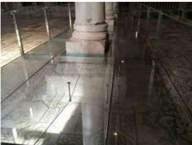
Fig.10 Glass footbridge with railings.
