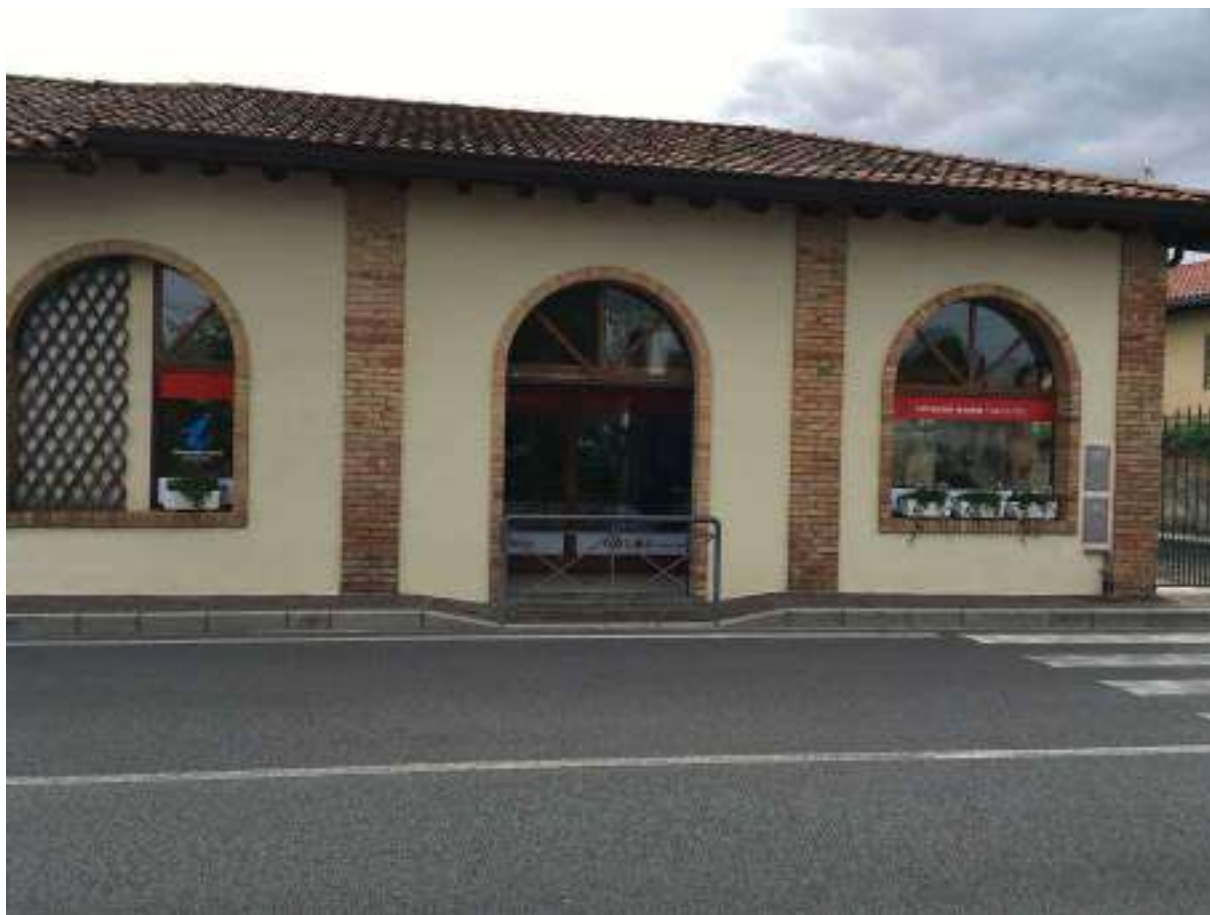
Fig.1 Offices of Infopoint of FVG of Aquileia.
