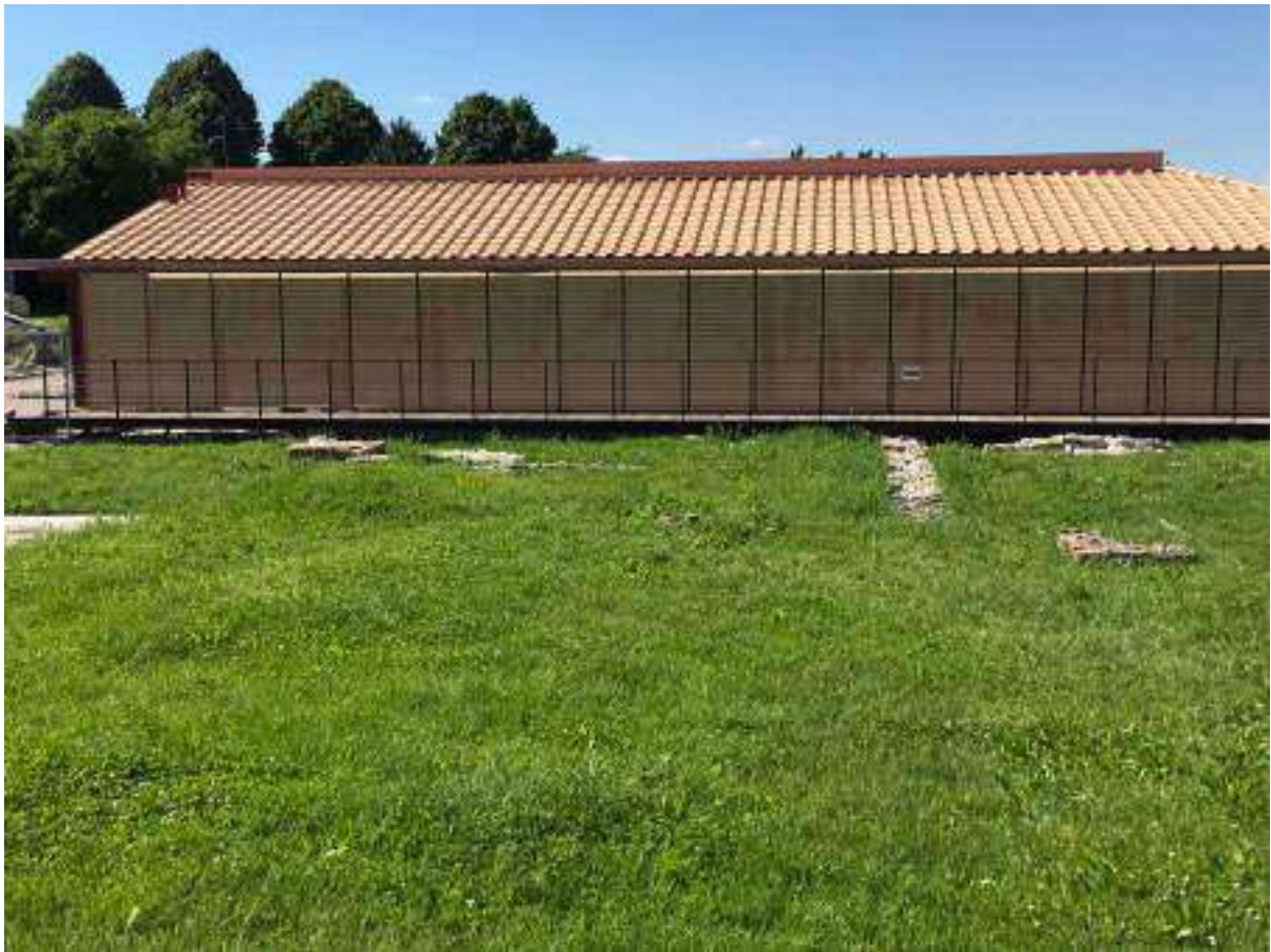
Fig.1 View of the new structure of the covering of the Fondo Cossar.
