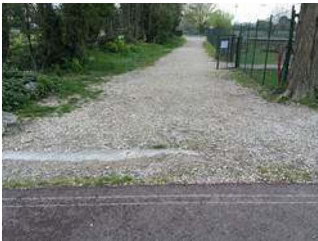
Fig.6 Gravel path connecting the cycling lane to the pavement.
