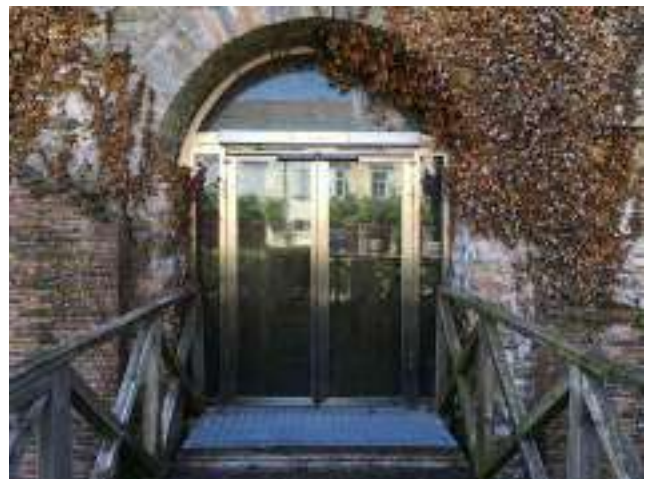
Fig.7 Door connecting with the interior.
