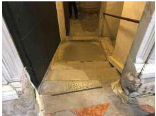
Fig.21 Ascent ramp from the crypt with railings.
