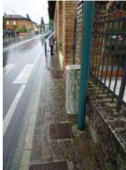
Fig.10 Pavement with a narrowing due to lamp-post and an energy-meter box.
