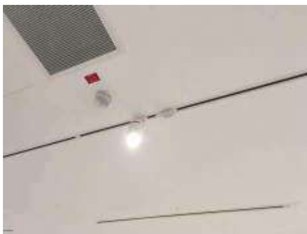
Fig.23 A beacon placed in the light support conduit.
