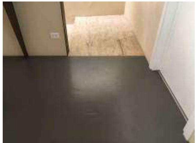
Fig.11 Chromatic contrast between the paving of the first floor and the stairway.
