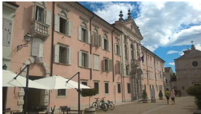
One of the buildings monitored (Gradisca d'Isonzo)
