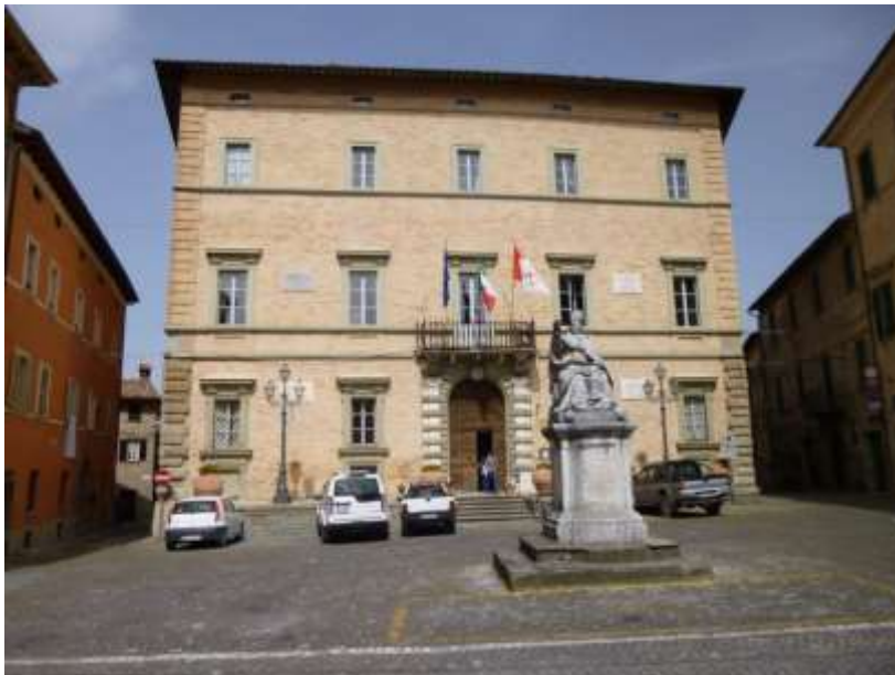
Figure 2. Example of Strategic Public Building monitored: Treia municipality. Masonry building built in the year 1773, last improvements made in 1973. Mansory typology: solid bricks and lime mortar masonry, horizontal structures truss with semirigid slabs and pushing and heavy roofing, foundation mat/plate.
