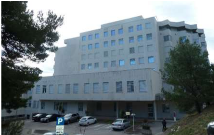
Figure 2. Dubrovnik Hospital – object D: seven (7) storey RC building.
