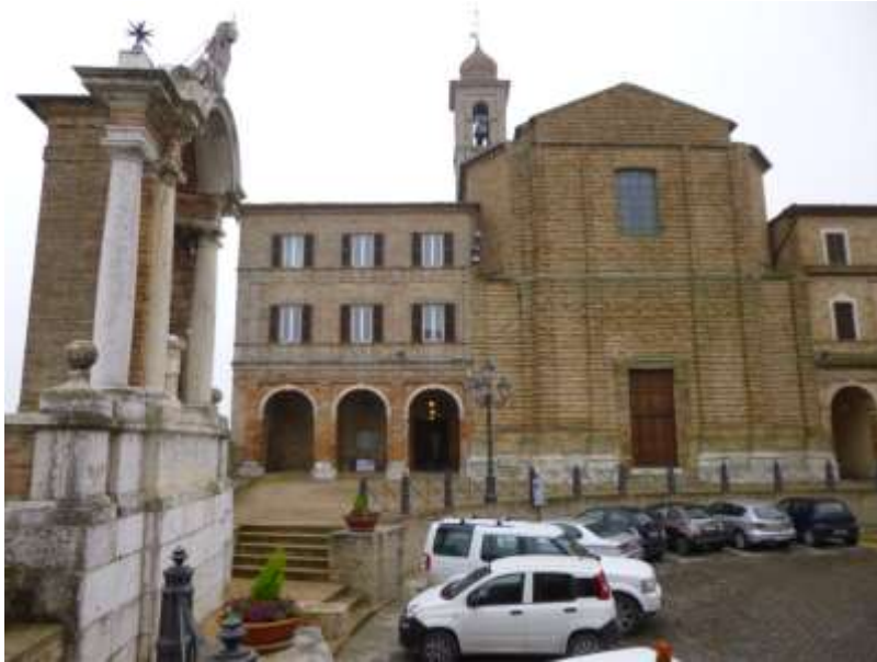
Figure 2. Example of Strategic Public Building monitored: Treia municipality. Masonry building built in the year 1773, last improvements made in 1973. Mansory typology: solid bricks and lime mortar masonry, horizontal structures truss with semirigid slabs and pushing and heavy roofing, foundation mat/plate.
